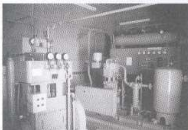
Central oxygen room. Left: Oxygen plant. Maintenance is very good for local standards. Right: Oxygen cylinders being refilled. The lateral stability of such cylinders should be improved by using devices designed to fit the cylinders to the ground while they are refilled.
