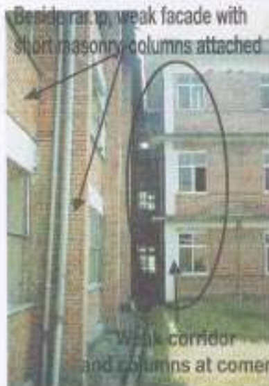
Left: Two blocks are rigidly connected with a weak corridor, which is likely to be crushed by strong ground shaking. The block on the right side is the out-patients, physiotherapy, and medical trainee centre block that has outer columns of 35 x 35 cm in size.
