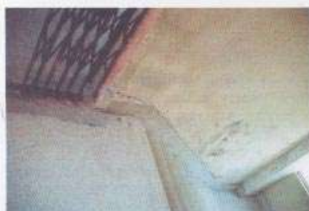
Cracks in pounding area between the "wedge" and the "L" building. Left: Top storey. Right: First storey.
