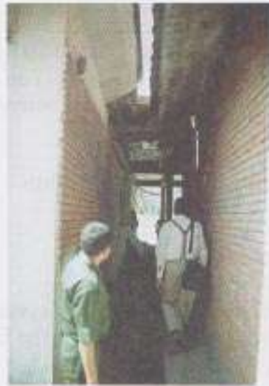
Left: Two blocks are rigidly connected with a weak corridor, which is likely to be crushed by strong ground shaking. The block on the right side is the out-patients, physiotherapy, and medical trainee centre block that has outer columns of 35 x 35 cm in size.
