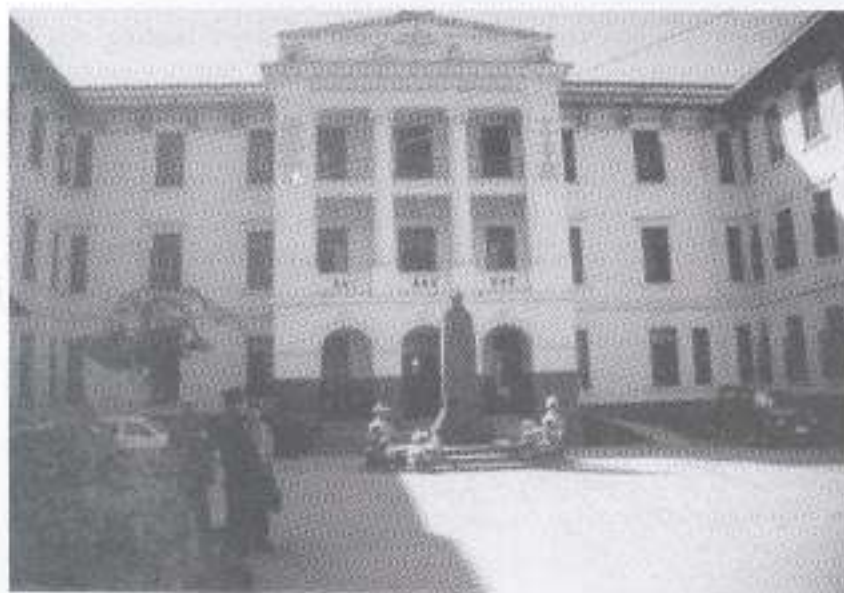
The Old Military Hospital building, which is considered to be able to withstand up to intensity MMI = IX earthquakes.
