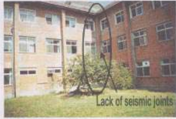
Left: Army Hospital main entrance. Right: One of the many re-entrant corners in the hospital. Decorative bricks cover the columns in the outer frames.
