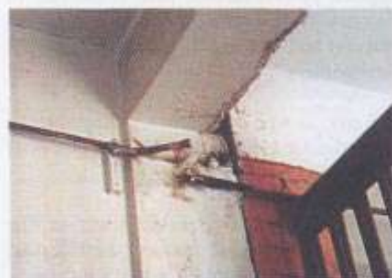
Left: Broken oxygen pipeline at pounding area of "L" building and the "wedge". Right: View from the "wedge".
